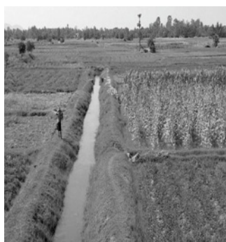
Vegetative planting and maintenance around small-scale natural irrigation canals
