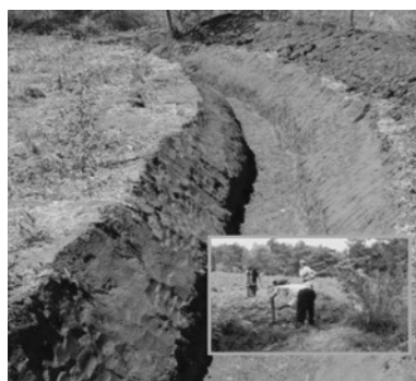
Contour trenching – water, moisture and soil conservation
